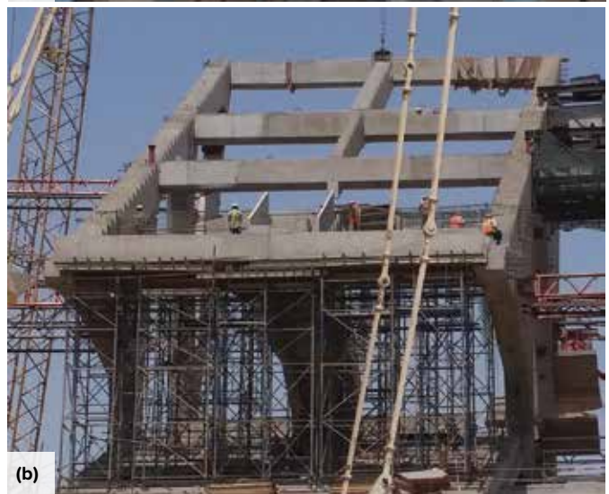
Fig. 14: Secondary radial beams (SRBs) were supported on circumferential beams: (a) view of a lower secondary beam; and (b) view of a completed bay
