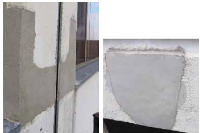
Fig. 8: Restoration of a 40-story reinforced concrete building in Philadelphia, PA, USA, in 2016. Spalled areas were repaired with a rubber-modified repair material. Repairs were to be subsequently covered with a polymer coating
