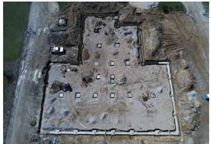
Fig. 1: Continuous and pad footings
