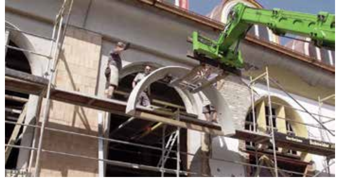
Concrete elements were assembled and installed at the project site
