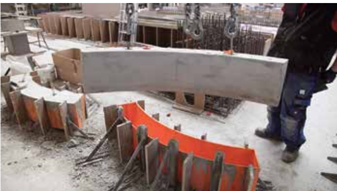
Production of a window frame element
