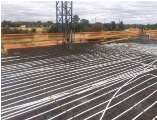
Fig. 7: A thermally activated building system (TABS) was installed in concrete slab floors and the roof to provide heating and cooling of the building
