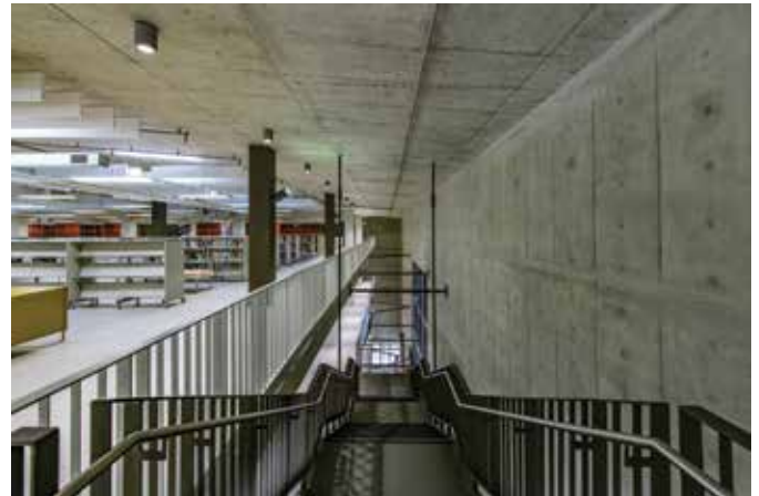
Fig. 5: Steel stairs are supported from above by tension rods from the roof
