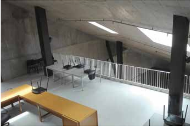
Fig. 6: The sloping roof slab created placing challenges
