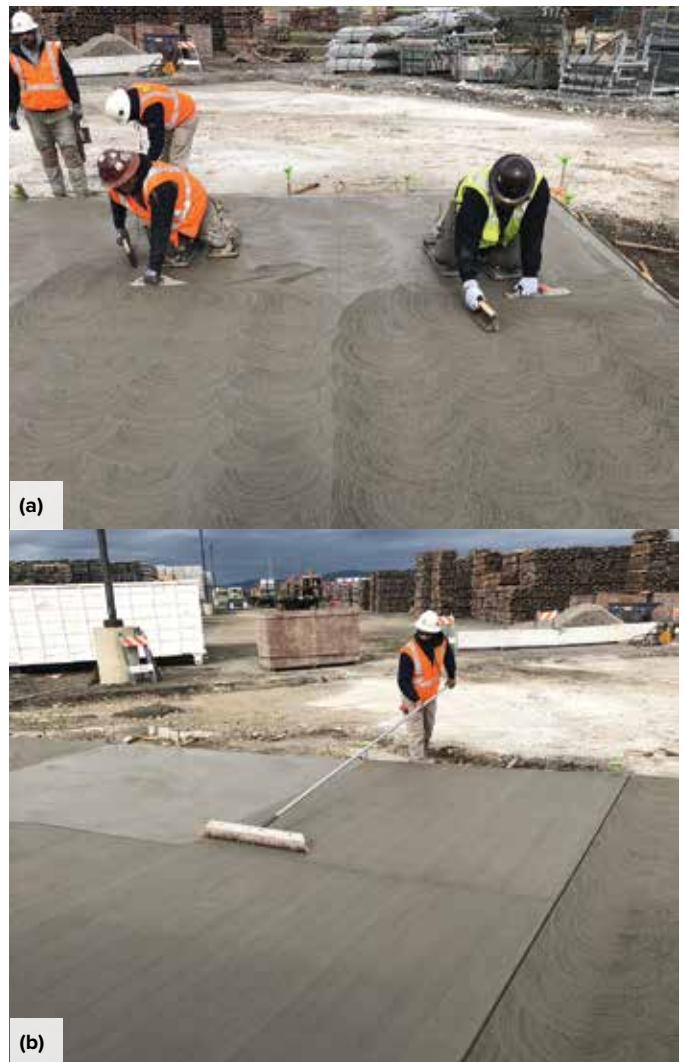
Fig. 1: Applying finishes to a test panel: (a) brush swirl finish; and (b) broom finish
