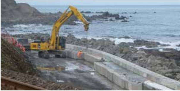
Fig. 1: Precast FRP-RC retaining walls at Kaikoura, New Zealand
