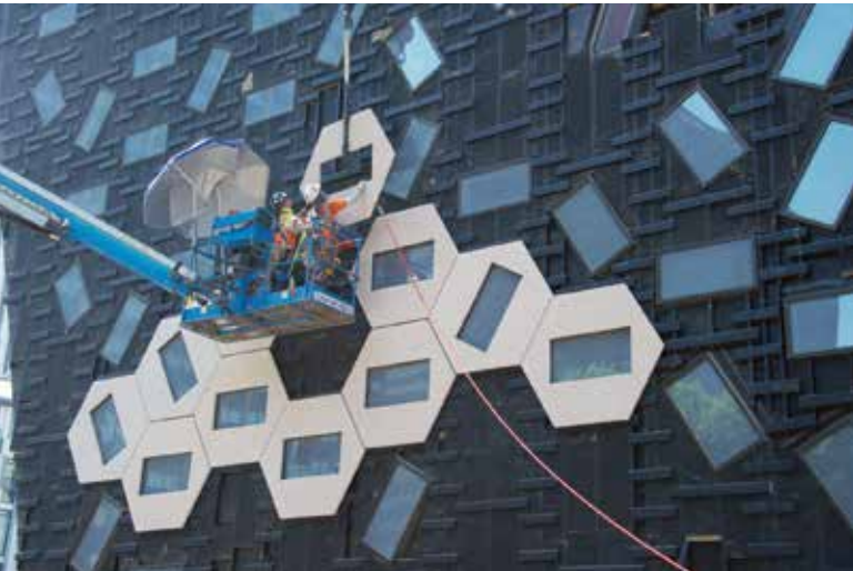
Fig. 5: GFRC panel installation (photos courtesy of Gary Leonard)
