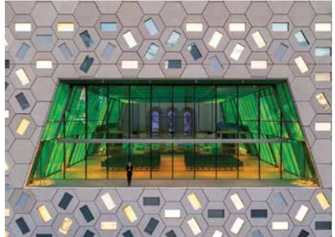
Fig. 3: The second-floor pavilion chapel outlines the temple dome through a vast window opening (image courtesy of OMA New York, photography by Jason O'Rear)
