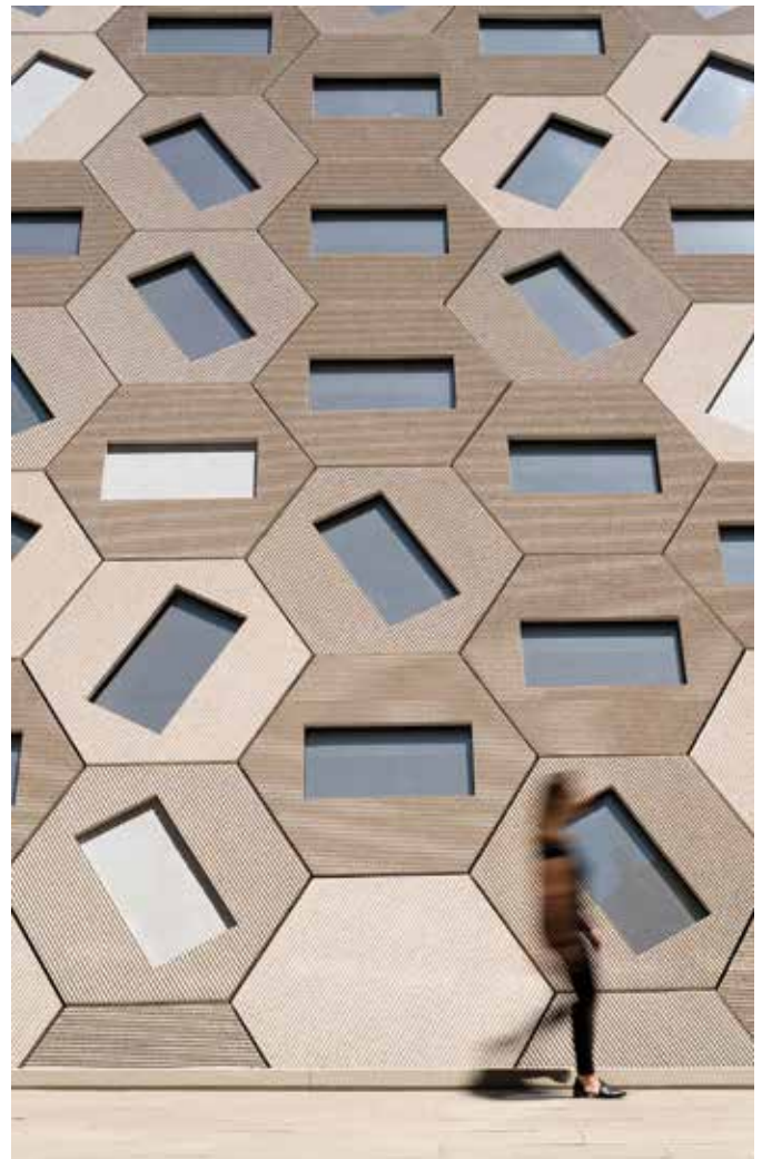
Fig. 4: Rectangular windows in adjacent hexagonal GFRC panels are rotated to create a dynamic building façade (image courtesy of OMA New York, photography by Jason O'Rear)
