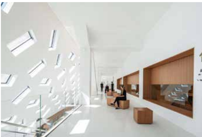
Fig. 2: The sloping design increases the building’s natural interior light (images courtesy of OMA New York, photography by Jason O’Rear)
