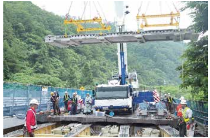
Fig. 4: Construction of a nonmetallic slab
