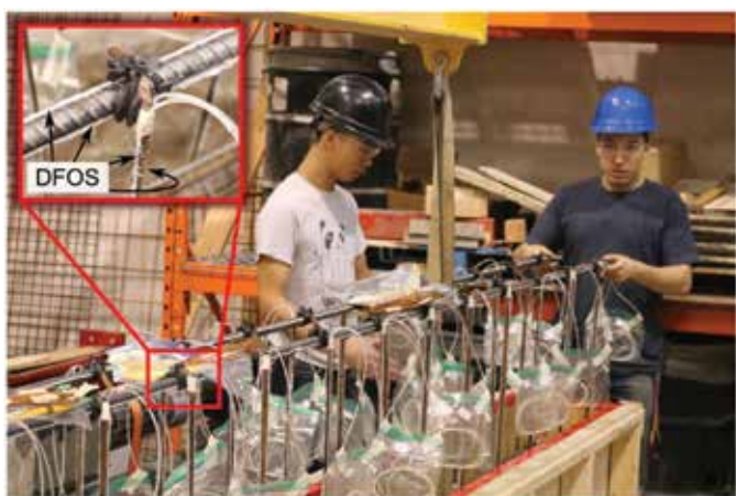
Fig. 3: Reinforcement cage of specimen JP-2 being lowered into the forms prior to concrete casting with DFOS bonded to the 20M reinforcement and 10M stirrups visible
