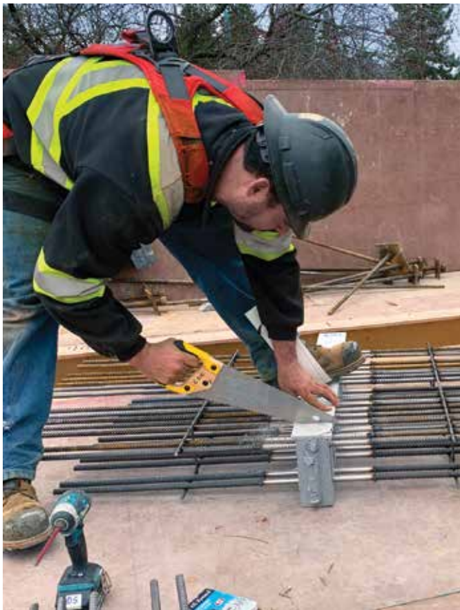
Fig. 2: A thermal break module may be cut with a handsaw if required
