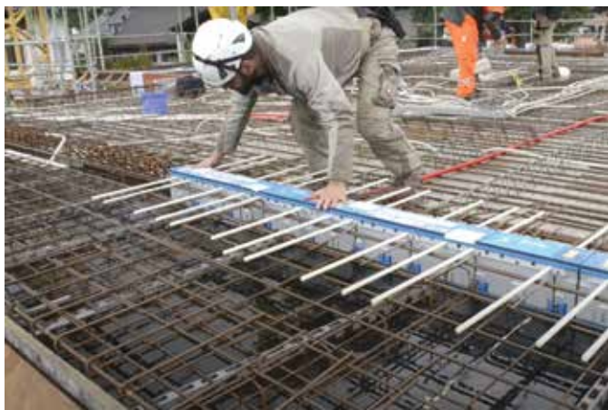
Fig. 1: Structural thermal breaks are relatively lightweight and can be installed by one person following the product's installation manuals and detailed illustrations. Alternate ends of each module are machined to provide tongue-and-groove joints and ensure a continuous and rigid installation. The blue top of each module is a protective polymer cap (firestops are also available). Note: The white bars in the photo are glass fiber-reinforced polymer (GFRP) bars
