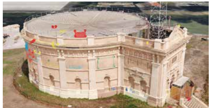
Fig. 9: Exterior damage can be highlighted on a 3-D model created using UAV photogrammetry
