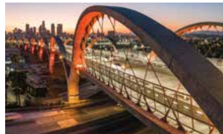
The Sixth Street Viaduct Replacement Project in Los Angeles, CA, USA, was a second-place winner in the Infrastructure category
