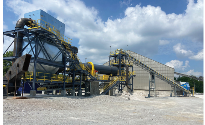
Additions to Heidelberg Materials' newly converted slag grinding facility in Speed, IN
