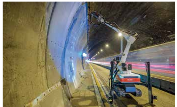
fischer BauBot construction robot working in a tunnel
