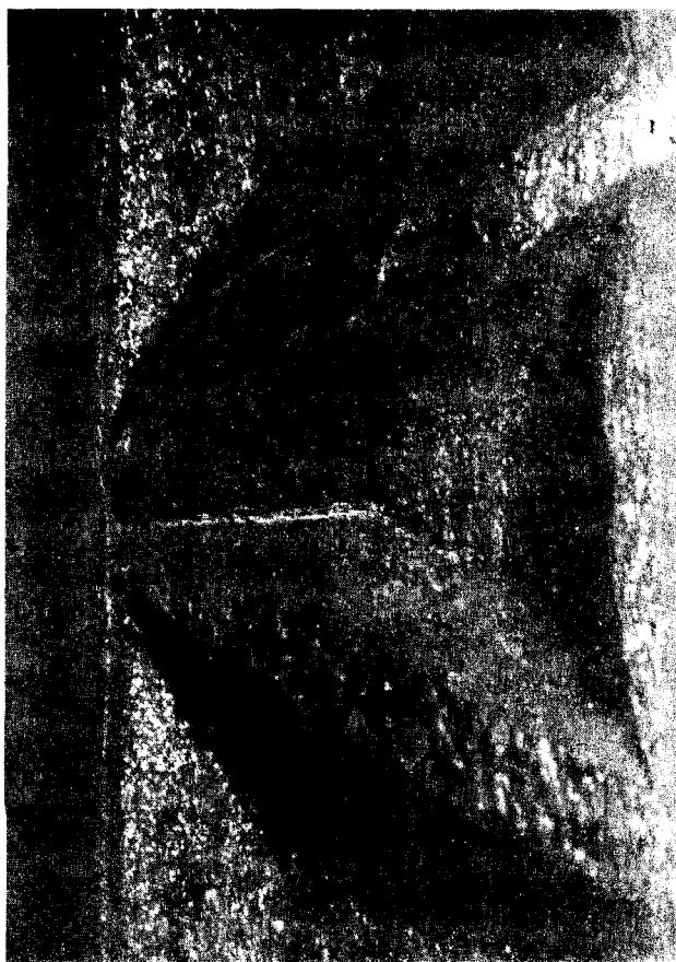
Fig. 6 — A 1/4-in. long crack in a #11 bar.
