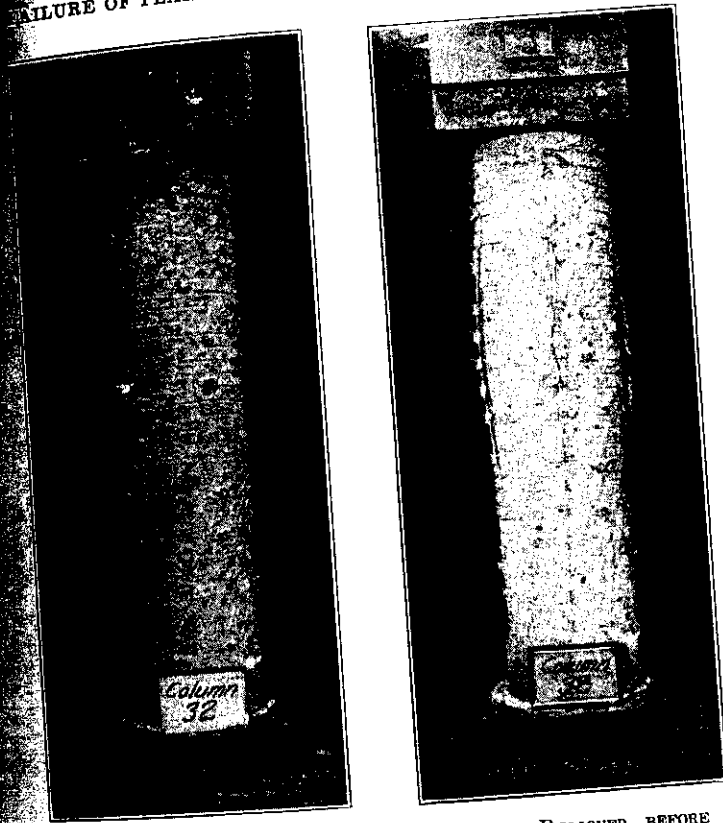
FIG. 7. VIEWS OF COLUMN 32 WITH SPIRALS REMOVED, BEFORE AND AFTER RETESTING
