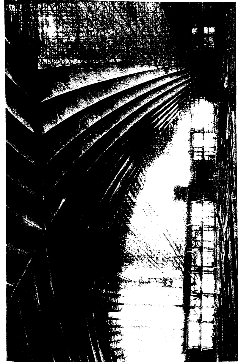
FIG. 12.—FORMS FOR EACH CONSTRUCTION STAGE, CONSTITUTING ONE-SIXTH OF THE ROOF, WERE SUPPORTED ON TUBULAR SCAFFOLDING.
