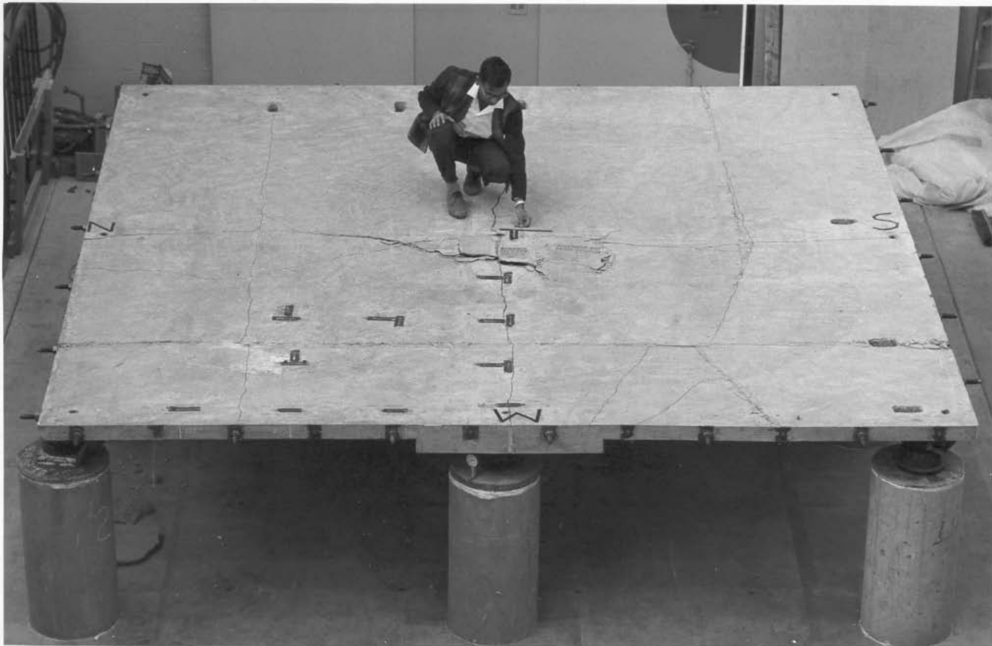
FIGURE 15: CRACK PATTERN ON TOP SURFACE AT FAILURE
