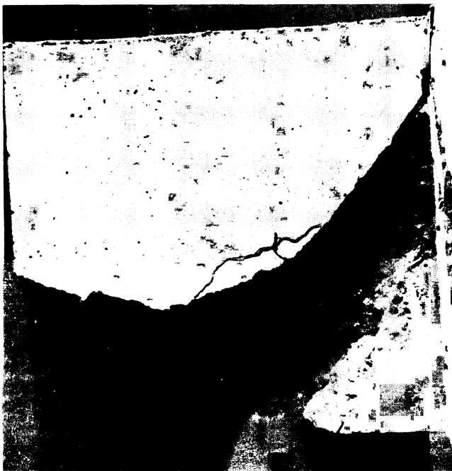
Fig. 9(b)—Appearance of failure zone in Pile Cap F after testing
