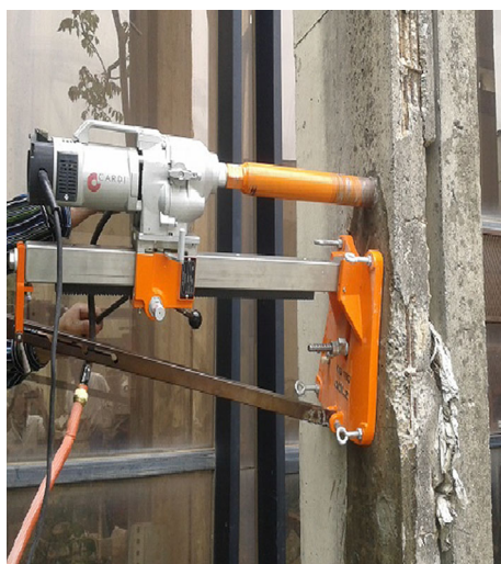
Fig. 21 Core drilling concrete.
