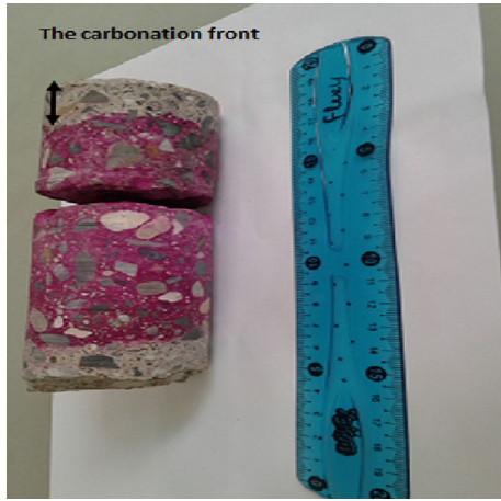
Fig. 19 The carbonation depth corresponding to the protected face.
