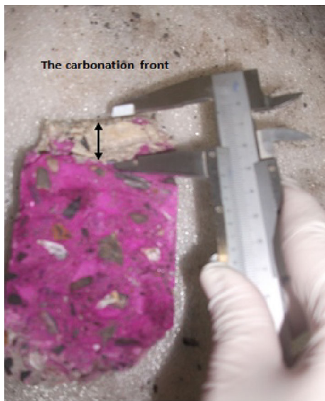
Fig. 20 The carbonation depth corresponding to the exposed and eroded face.
