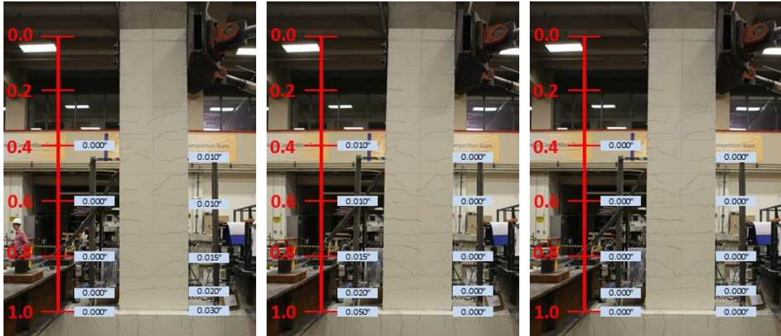
Figure C-17: Measured Crack Widths at Drift Ratio of 0.9% – Specimen SBL100
