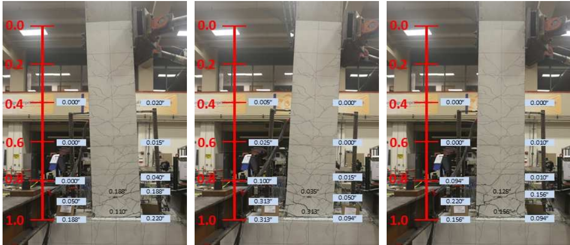
Figure C-15: Measured Crack Widths at Drift Ratio of 4.85% – Specimen SBH100
