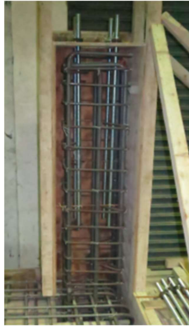
(b) Placement of Threaded Rods
