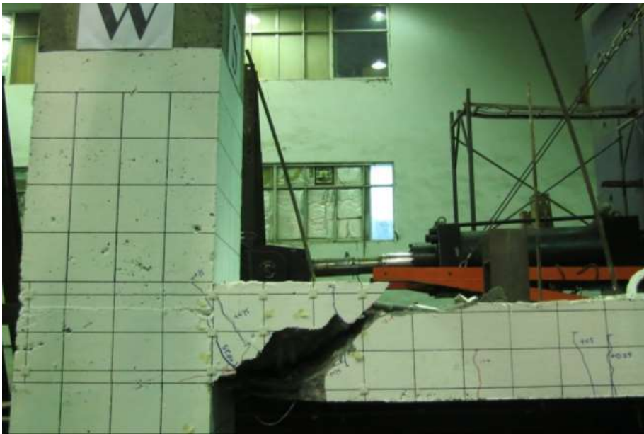
(b) After Loose Concrete Removal
