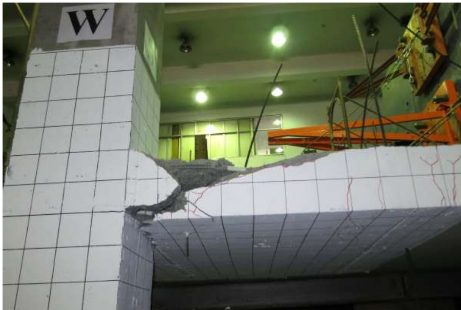
(b) After Loose Concrete Removal
