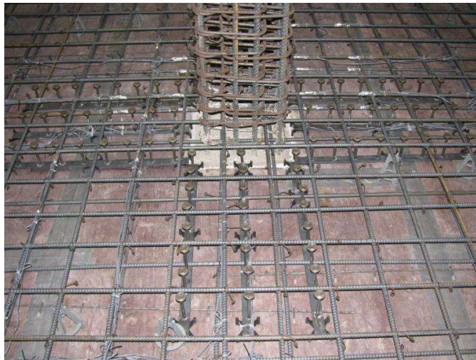
(b) Headed Shear Studs
