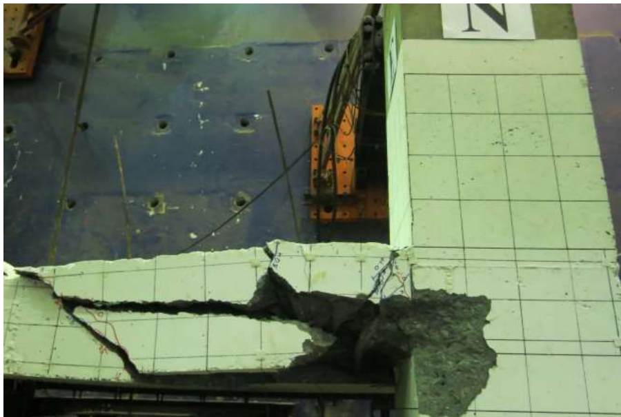
(b) After Loose Concrete Removal
