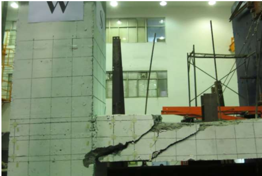
(b) After Loose Concrete Removal
