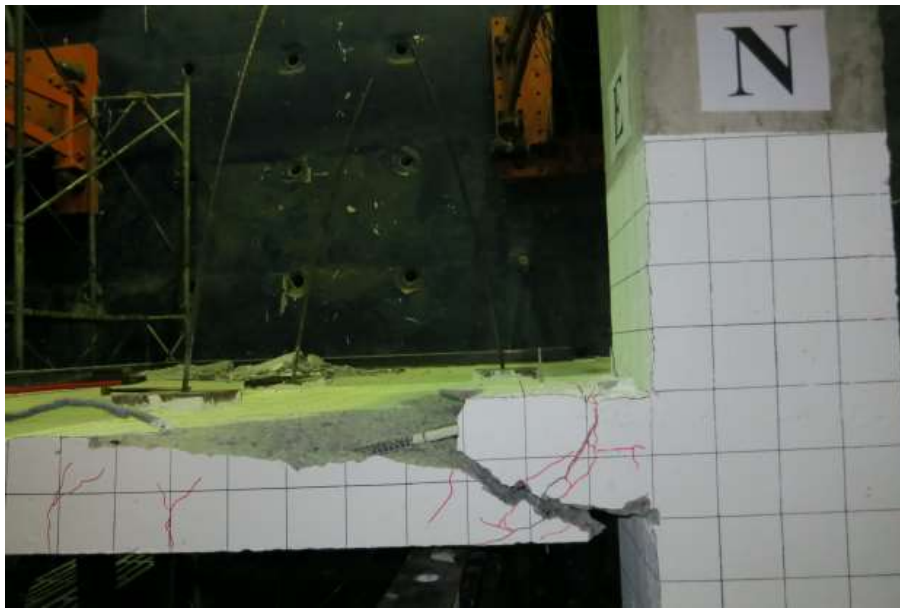
(b) After Loose Concrete Removal
