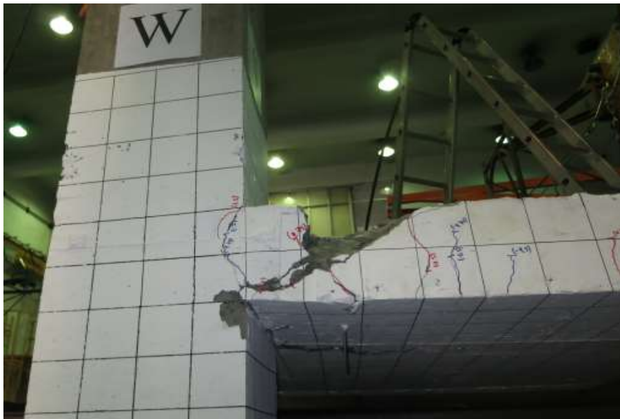
(b) After Loose Concrete Removal
