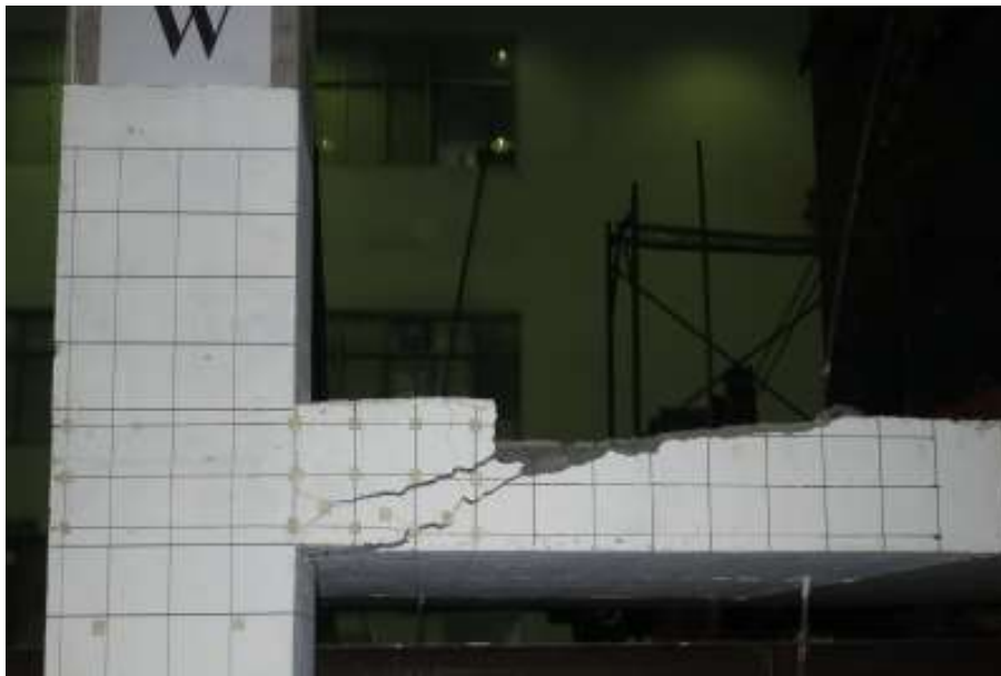
(b) After Loose Concrete Removal
