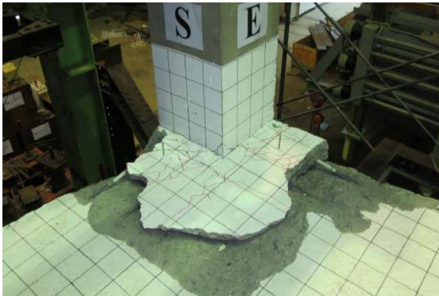
(b) After Loose Concrete Removal
