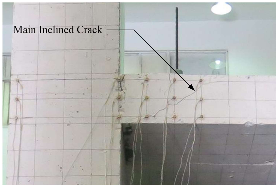
Fig. 4.51– Crack Pattern on the West Slab Face of Specimen R3 at 1.75% Drift
