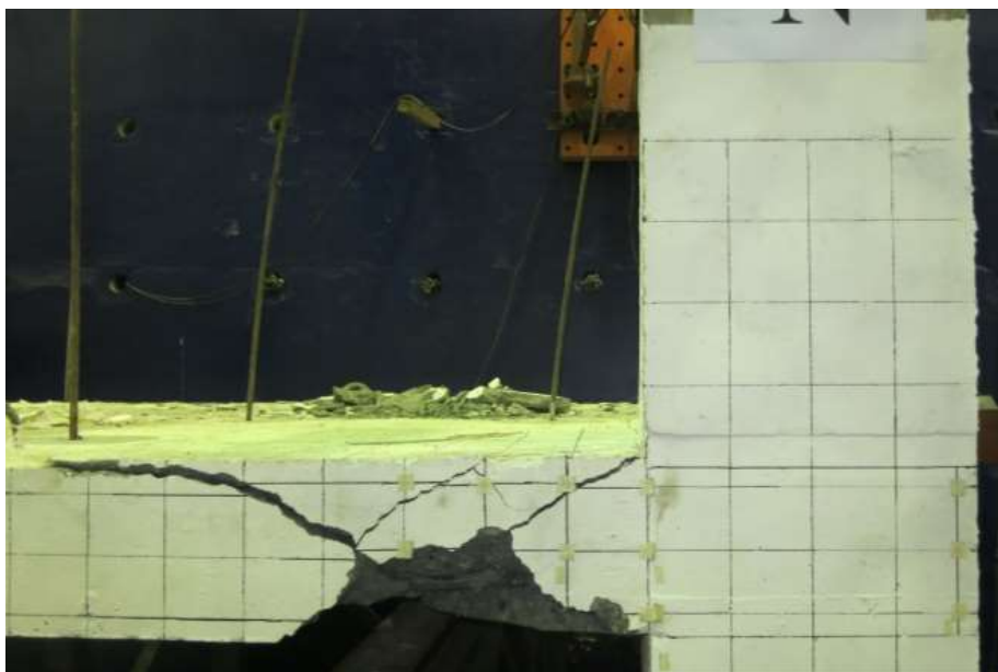
(b) After Loose Concrete Removal
