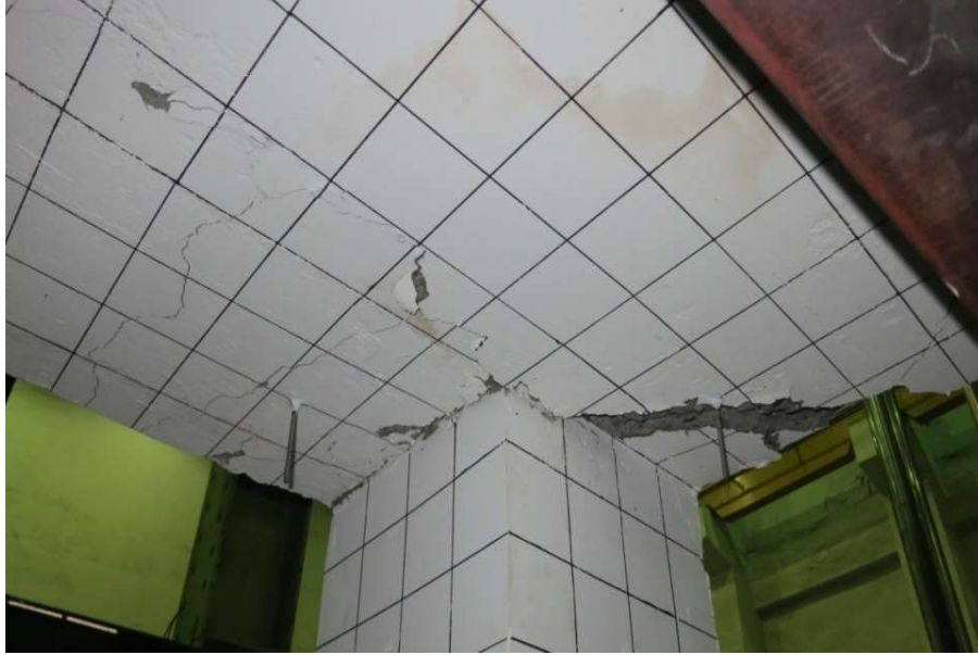
Fig. 4.21 – Slab Bottom Surface of Specimen G1 Near the Connection at Failure
