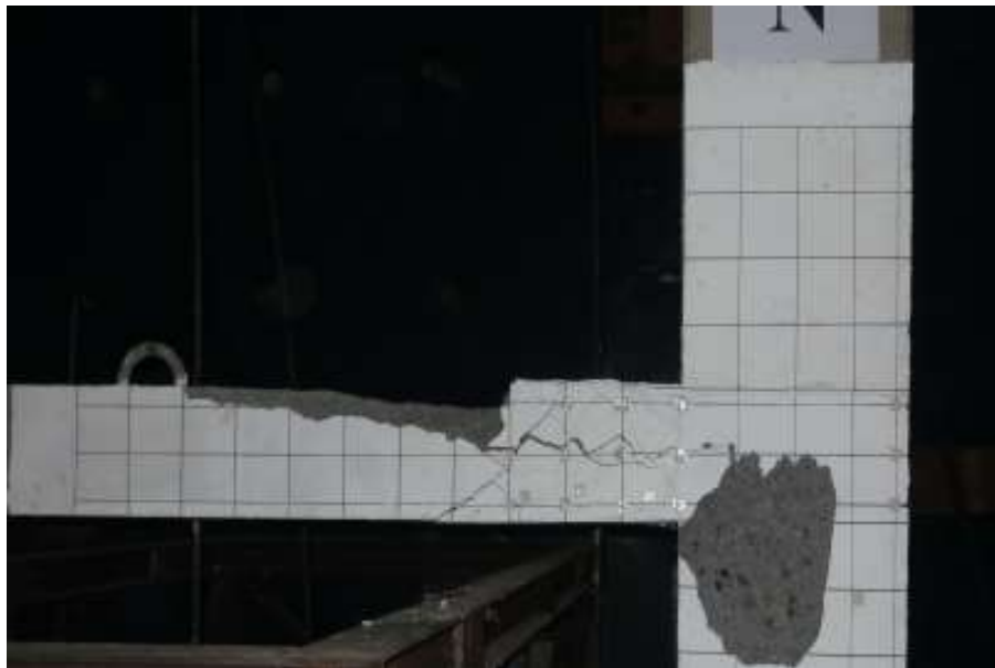
(b) After Loose Concrete Removal
