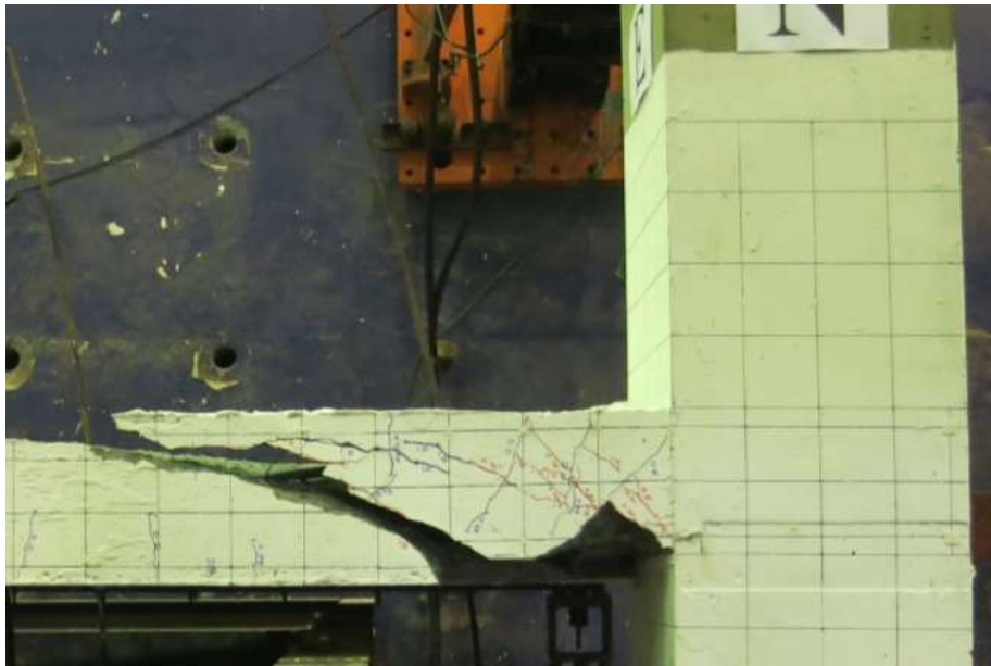
(b) After Loose Concrete Removal
