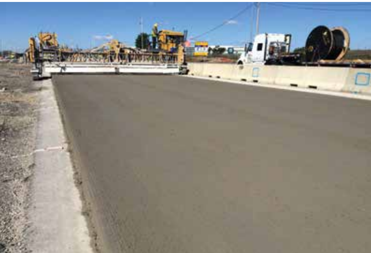
Jane Addams Memorial Tollway (I-90) Rebuilding and Widening project credits: Illinois Tollway, Owner/Engineer; Walsh Construction Company, Contractor; and Terrell Materials Corporation, Concrete Supplier
