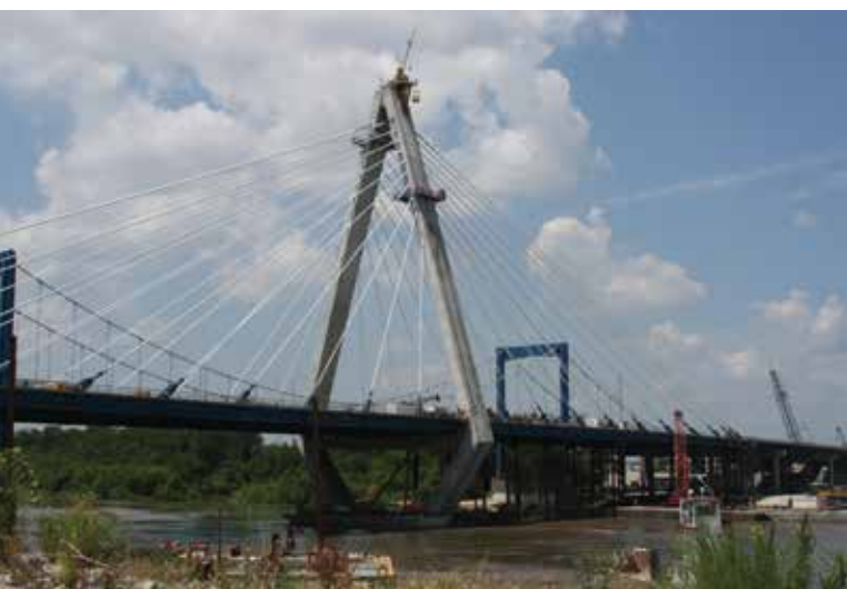
Christopher S. Bond Bridge project credits: MoDOT, Owner; Parsons Corp., Engineer; Paseo Corridor Constructors (a partnership of Massman Construction Co, Clarkson Construction Co, and Kiewit Construction Co), Contractor; and Fordyce Concrete, A Division of Ashgrove Materials Corp, Concrete Supplier
