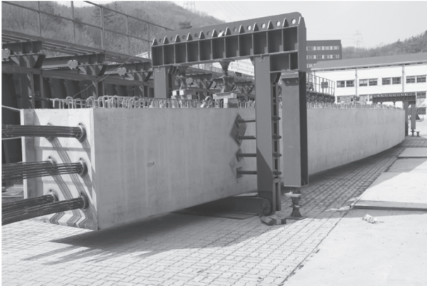
Fig. 2 Lift device for preventing over-turning rotation of a curved girder.
