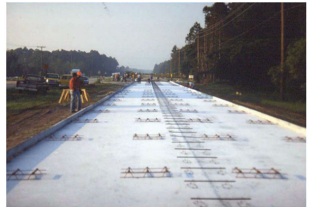
(b) Special dowel arrangement
