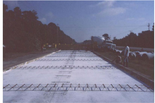
(a) Standard dowel arrangement
