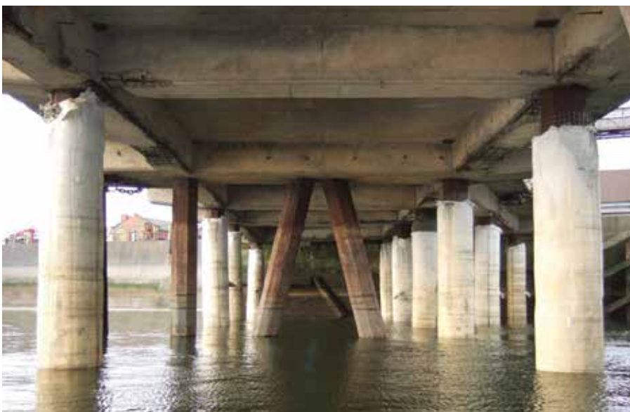
Fig. 4: Sleeve formwork can be used to form jackets for repair of damaged piles 13
