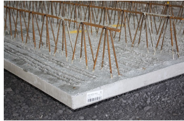
Fig. 3 Precast concrete lattice girder plank.
