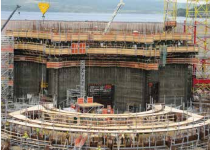
Fig. 3: Slipforming of the Hebron GBS, Newfoundland and Labrador, Canada
