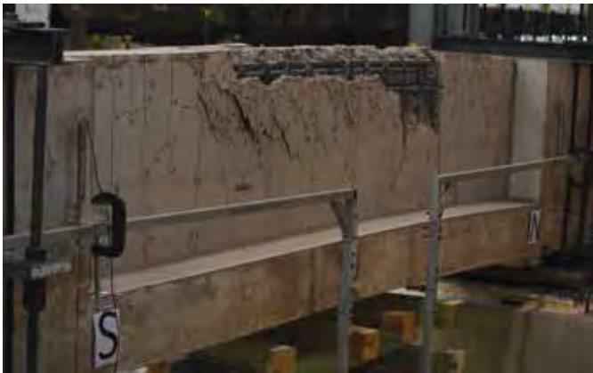
Fig. 7: Splice failure in test beam
