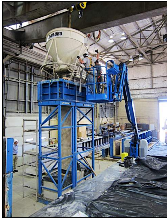
Figure 10: Column casting process
