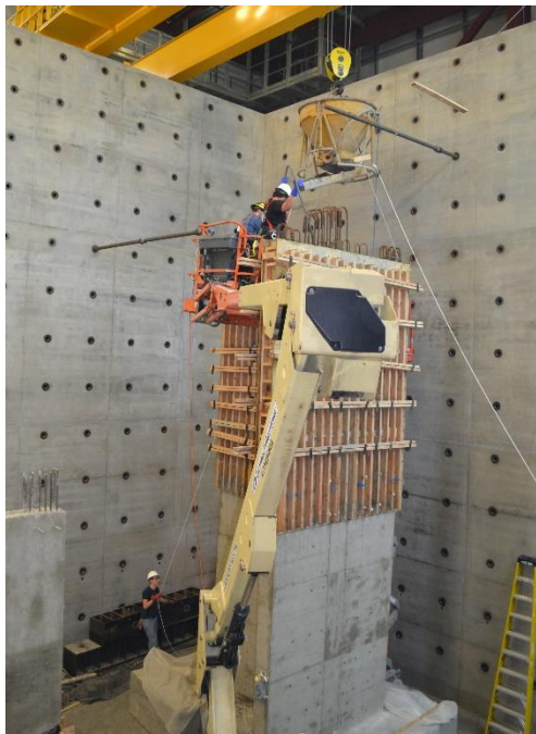
Figure 24 – Lift 2 casting (T3)
