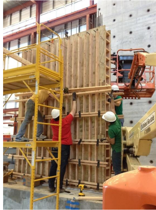
Figure 23 – Lift 1 formwork assembly (T1)
