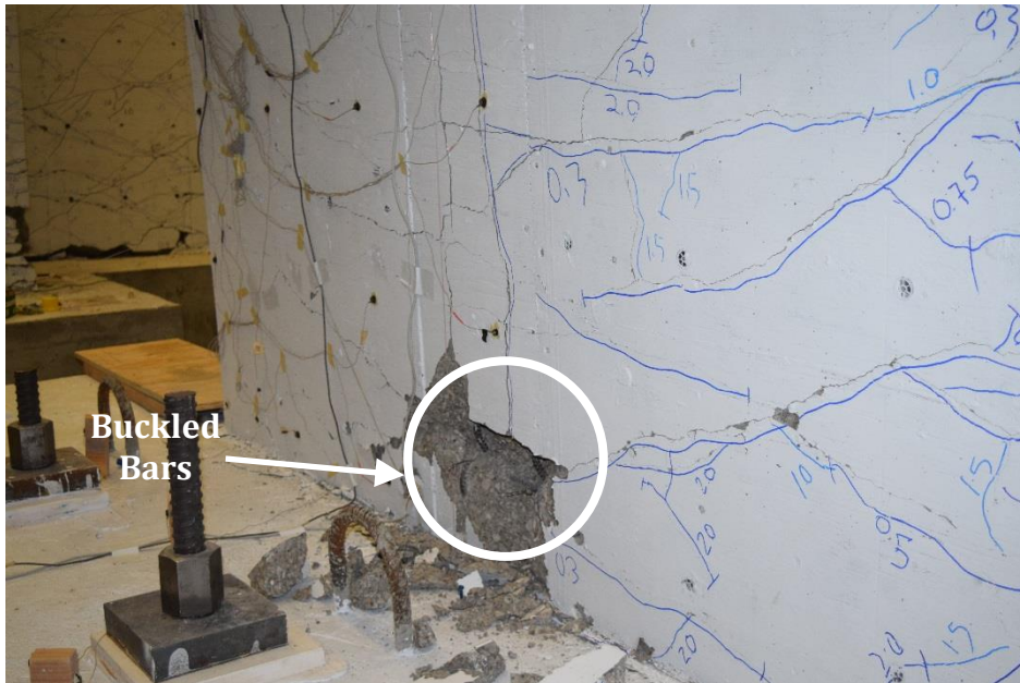
Figure 71 – Wall T4 with bar buckling in unconfined flange during second cycle to 3% drift ratio (stem in tension)
