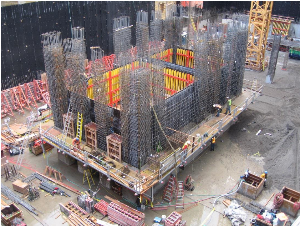
(b) Base of a tall core-wall building
