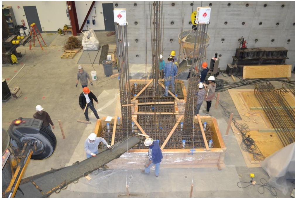
Figure 20 – Casting of base block for T1
