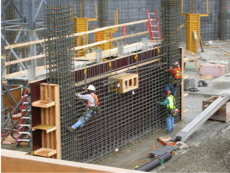
(a) Base of a medium-rise wall building
