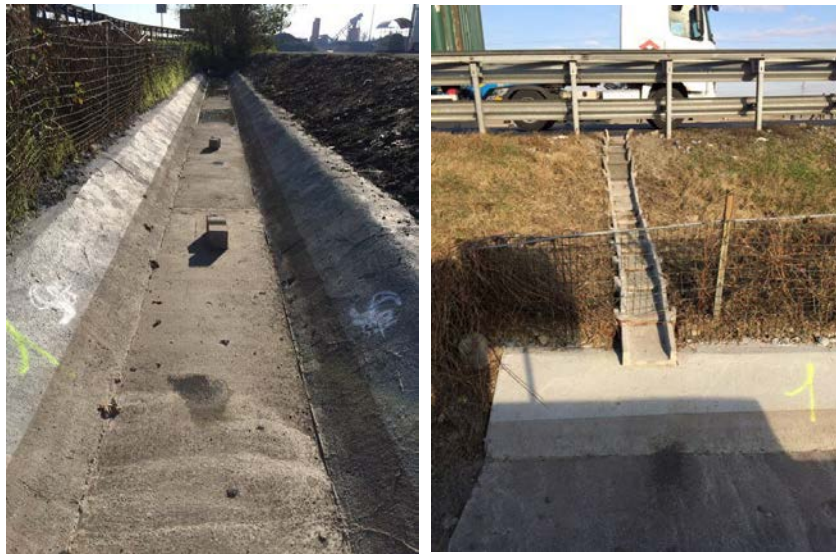
Figure 4 – Culvert (left) and a lateral ditch for water collection from roadway (right)
