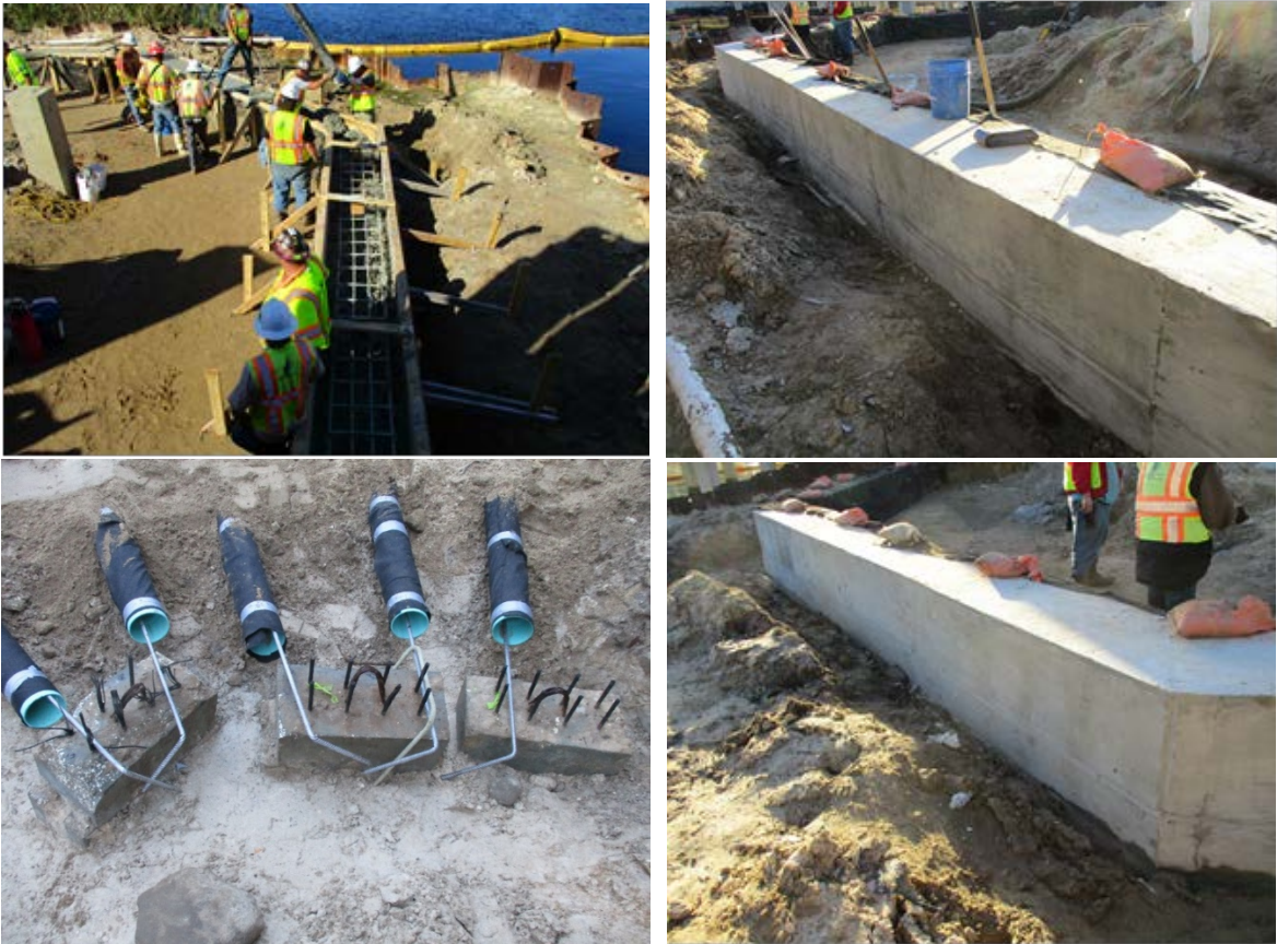
Figure 15 – Bulkhead cap concrete placement and final product
