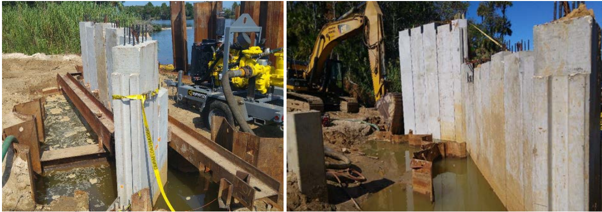
Figure 12 – GFRP-RC sheet pile retaining wall
