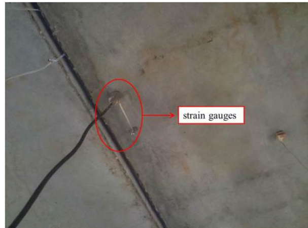
(b) Strain gauges on the bottom flange of the girder
