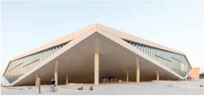
The building's west and south façades thrust upward to create a dramatic cantilever over the main entry to the library
