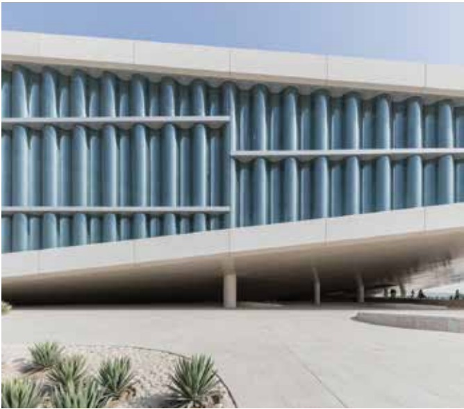
Deeply corrugated glazing provides filtered light for reading and study
