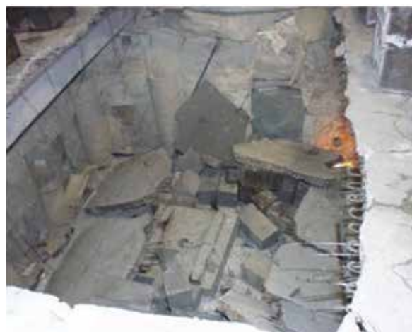
Fig. B: Photo from p. B-3 of Reference 19. The original caption states: “Load Collapse At 3 Min 55 Sec After Fire Exposure Ended”
