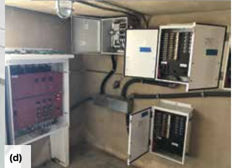
Fig. 6: ICCP system features: (a) anode and isolation from low-cover reinforcing bar; (b) grouted anode slots; (c) balcony deck as finished with vertical conduit (photo taken 2010); and (d) control and power system components (May 20, 2019)
