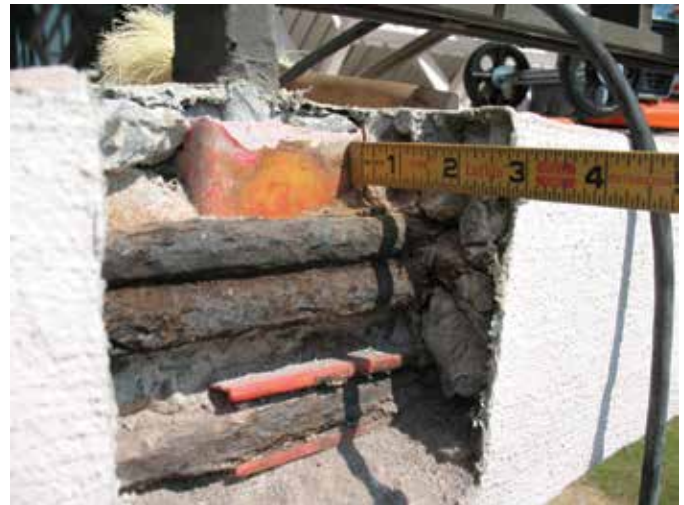
Fig. 2: Example of test excavation during 2007 assessment
