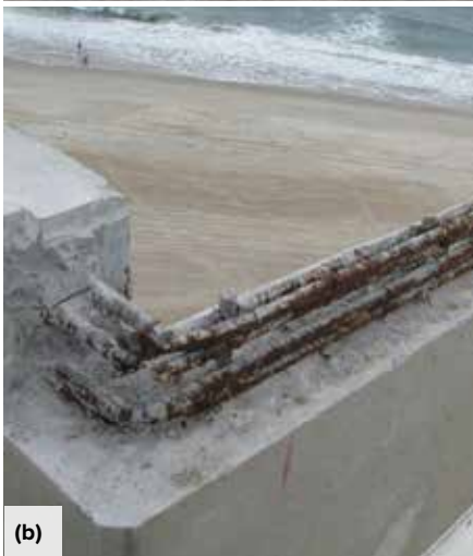
Fig. 6: ICCP system features: (a) anode and isolation from low-cover reinforcing bar; (b) grouted anode slots; (c) balcony deck as finished with vertical conduit (photo taken 2010); and (d) control and power system components (May 20, 2019)
