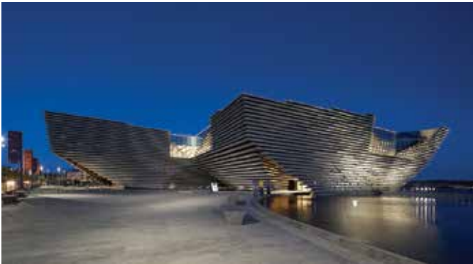
Fig. 4: From a distance, the building looks like a sturdy ship (photo courtesy of HUFTON + CROW)
