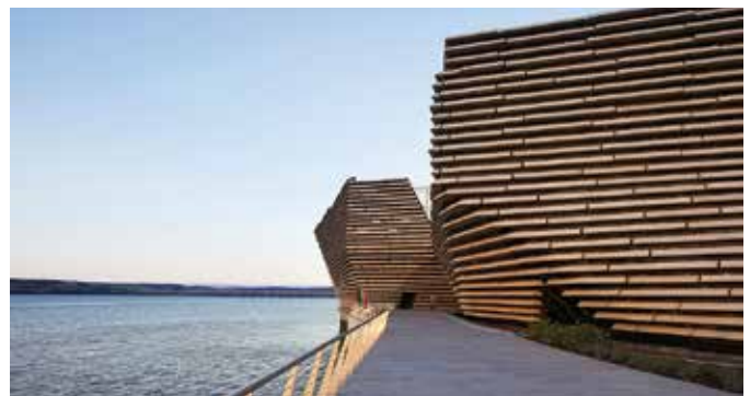
Fig. 3: The striated building façade invokes images of the Scottish coastline cliffs (photo courtesy of HUFTON + CROW)
