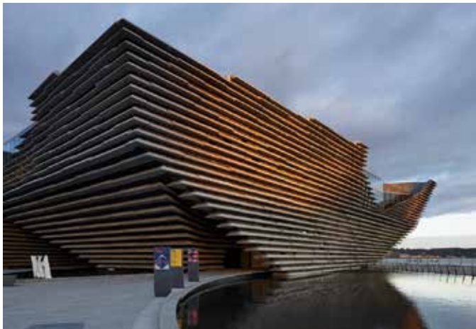
Fig. 10: The cliff face appearance of the building's exterior was executed with 2429 precast concrete panels
