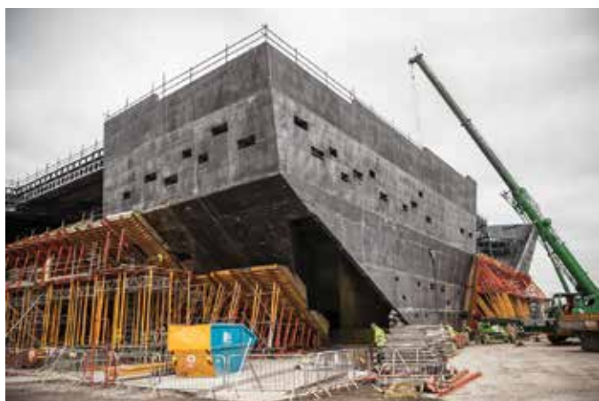
Fig. 8: Façade walls remained propped until the internal floor plates, beams, and slabs were fully tied into the structure and the concrete had reached design strength
