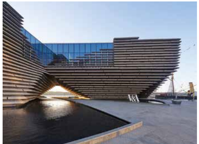
Fig. 2: The building has the form of two inverted pyramids (photo courtesy of HUFTON + CROW)
