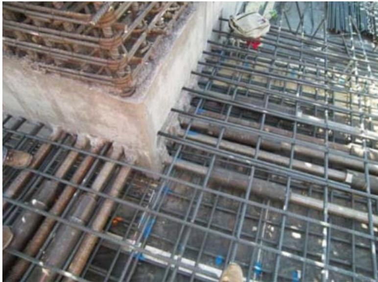
**Appendix A-15: Photograph showing reinforcement congestion at a diaphragm-to-wall connection. Bigger reinforcing bars are collectors. Smaller reinforcing bars are shear friction reinforcement [20].**
