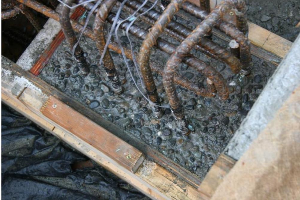
**Figure 3.6: Photograph of a surface treated with surface retarder.**
