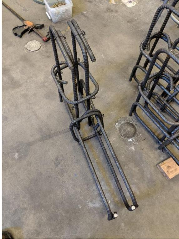
**Appendix A-6: Half of the reinforcement cage constructed**
