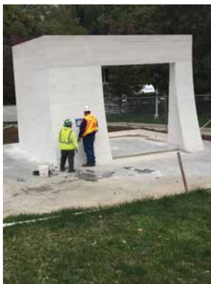
Fig. 17: Visual mockups were used to test concepts for formwork, form ties (steel or fiber composite), jointing, embed placement, and patching
