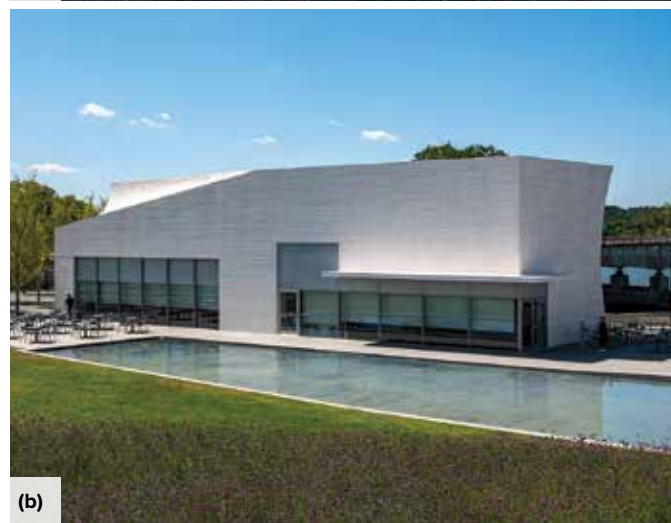
Fig. 10: A conical roof slab is a prominent feature of the River Pavilion. In contrast to the conical slab at the Welcome Pavilion, this feature was placed using a single layer of manually finished white concrete: (a) an interior view; and (b) an exterior view
