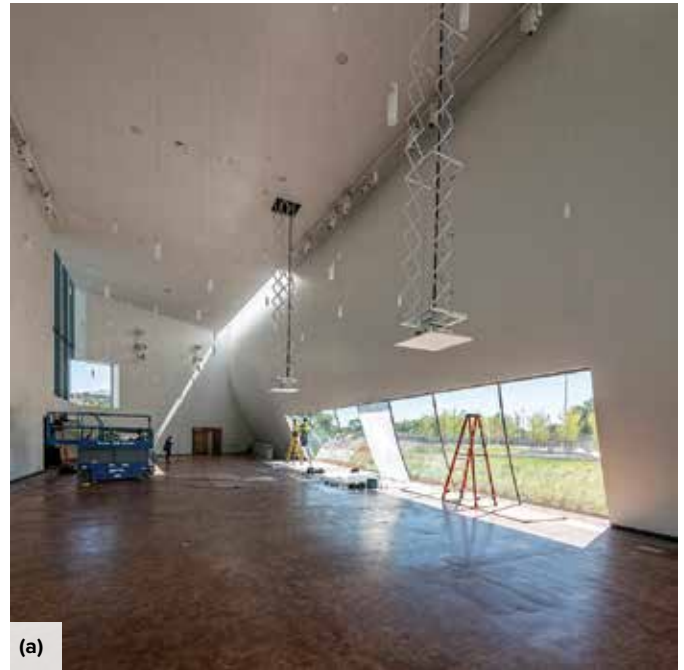
Fig. 6: The conical slab comprises a gray structural concrete layer, a roofing membrane, and a white exterior layer. The form was achieved using both formed concrete and shotcrete placements.
