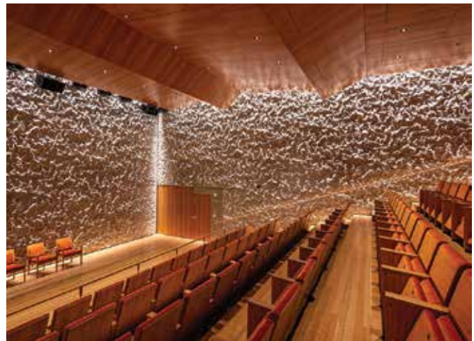
Fig. 13: The Justice Forum auditorium also includes crinkle concrete walls. The steps, door openings, and corner reveals created challenges in laying out the liner panels and forming the bulkheads, as a running bond pattern was required to avoid creating a discernable repeating pattern in the crinkle finish. Further, many of the walls had crinkle liner on one side and board-form finish on the other
