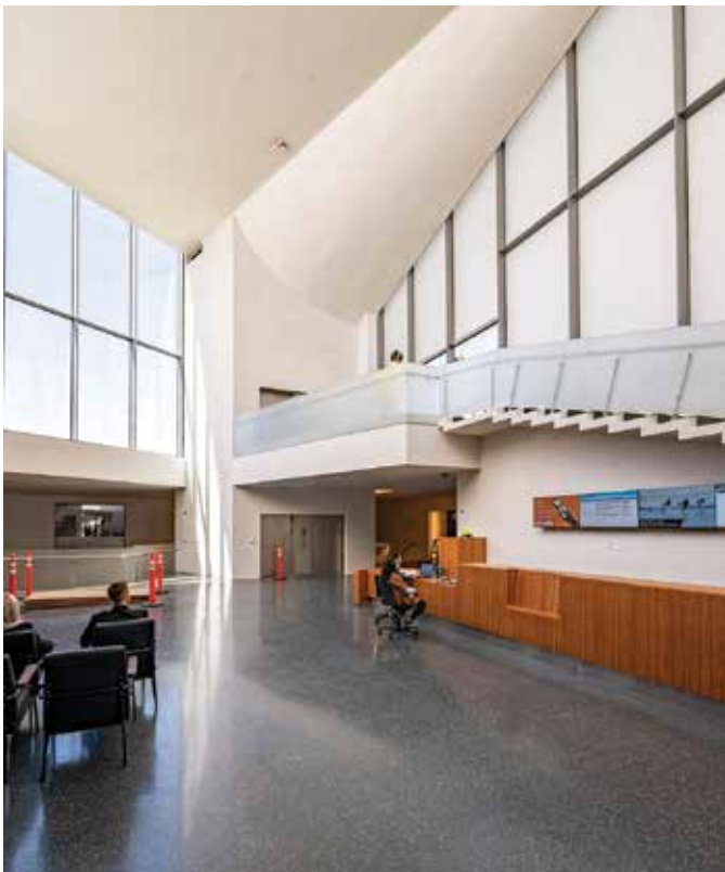
Fig. 3: A conical roof slab and cantilevered concrete stairs provide distinctive features in the atrium of the Welcome Pavilion
