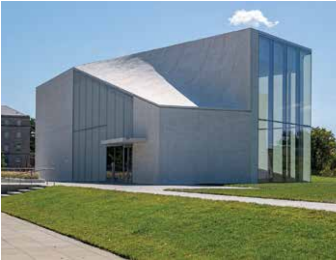
Fig. 6: The conical slab comprises a gray structural concrete layer, a roofing membrane, and a white exterior layer. The form was achieved using both formed concrete and shotcrete placements.
