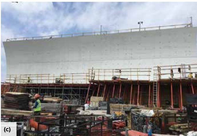
Fig. 9: The curved “feature” wall of the Skylight Pavilion required an extremely complex formwork system: (a) the initial formwork towers above the site, adjacent to the tower crane; (b) the tongue-and-groove board finish was especially challenging to create on the curved surface; (c) uniform tie spacing was required; and (d) the scale of the wall is made clear by this photo of the crew commemorating the final placement of the wall concrete
