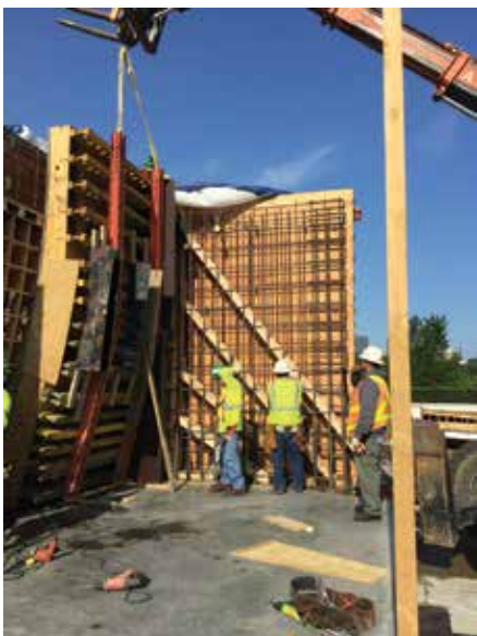
Fig. 17: Visual mockups were used to test concepts for formwork, form ties (steel or fiber composite), jointing, embed placement, and patching
