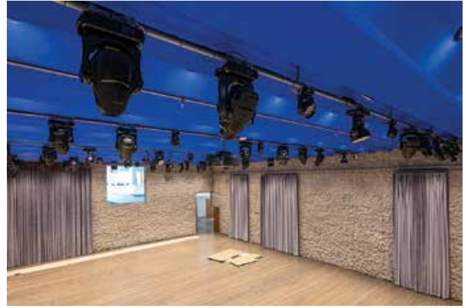
Fig. 12: Studio K is a multipurpose room that takes its name from the late president’s last initial. The space includes acoustic “crinkle” concrete walls and a sawtooth concrete ceiling with integral light fixtures. The concrete slab soffit profile was cast to match the form of the blue covering. Although this slab supported the green roof and was post-tensioned, it did not include void formers
