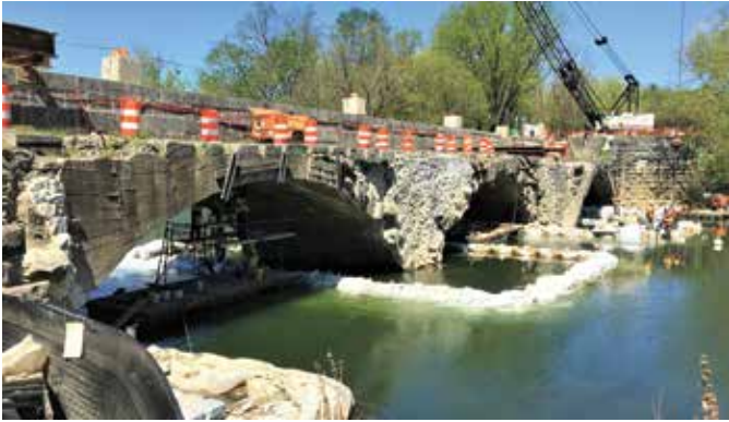
Reinforcing piers and abutments
