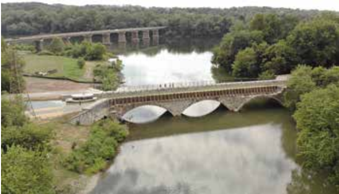
Conococheague Aqueduct after construction
