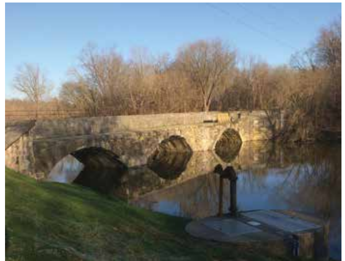
Conococheague Aqueduct before renovation
