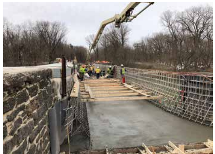
Base slab placement (photo courtesy of Thomas, Bennett & Hunter, Inc.)
