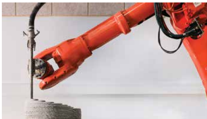
3D concrete printing
