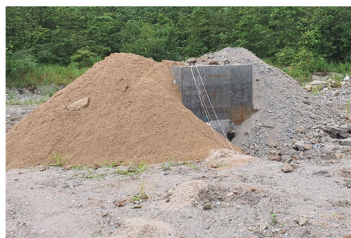
(b) High-strength concrete structure before explosion
