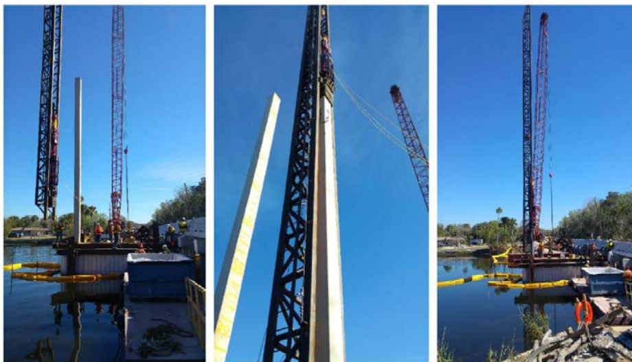
Figure 10 – CFRP-PC bearing piles
