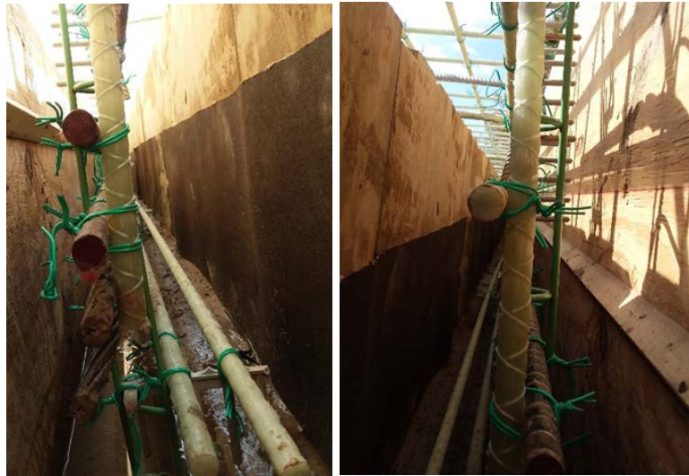
Figure 14 – Sample bars in test blocks before concrete casting
