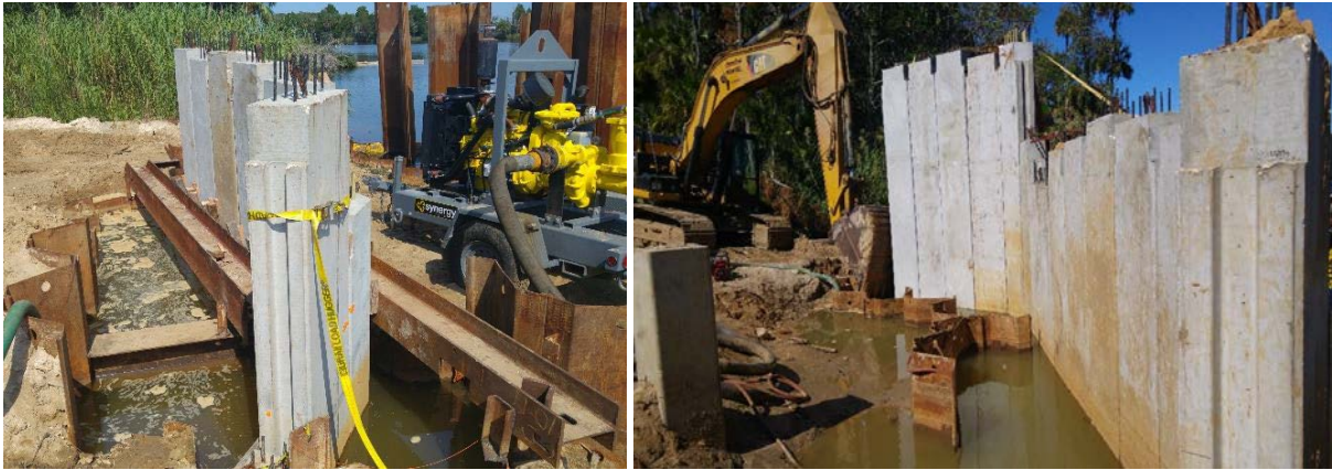
Figure 12 – GFRP-RC sheet pile retaining wall
