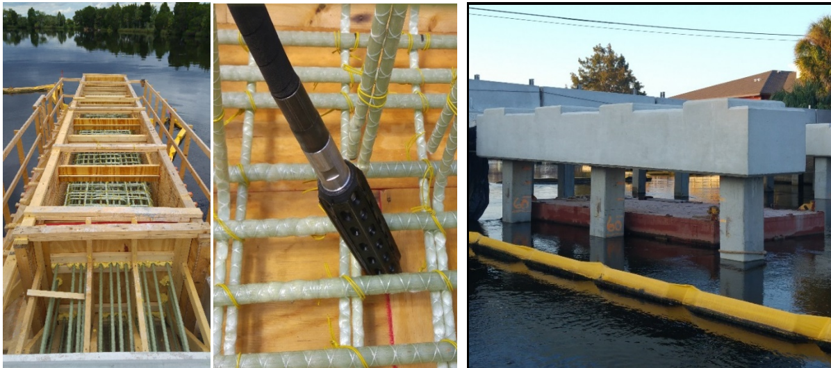
Figure 11 – GFRP-RC bent caps
