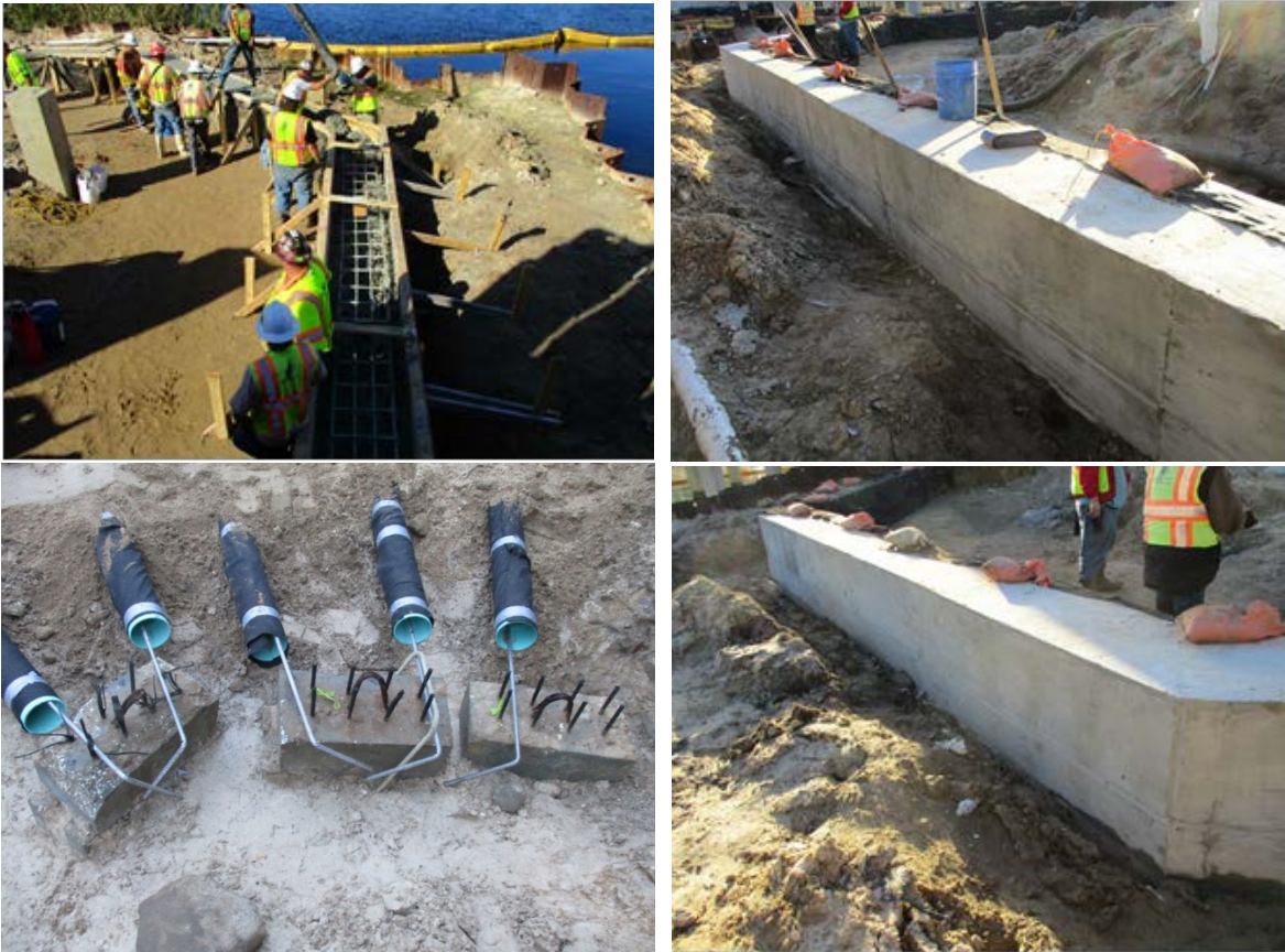
Figure 15 – Bulkhead cap concrete placement and final product
