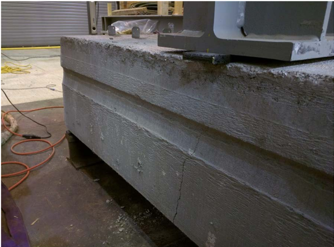
Figure B19 - Test span S2-F1-66-2.3
