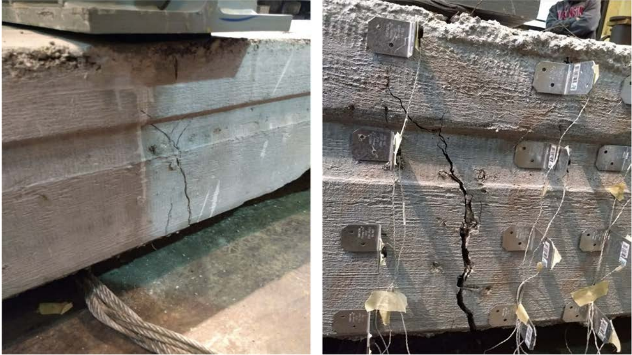
Figure B30 - Test span S2-F2-50-3.0
