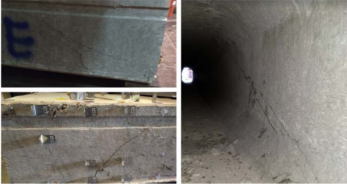
Figure 12- Typical web cracking for test spans in Series 1
