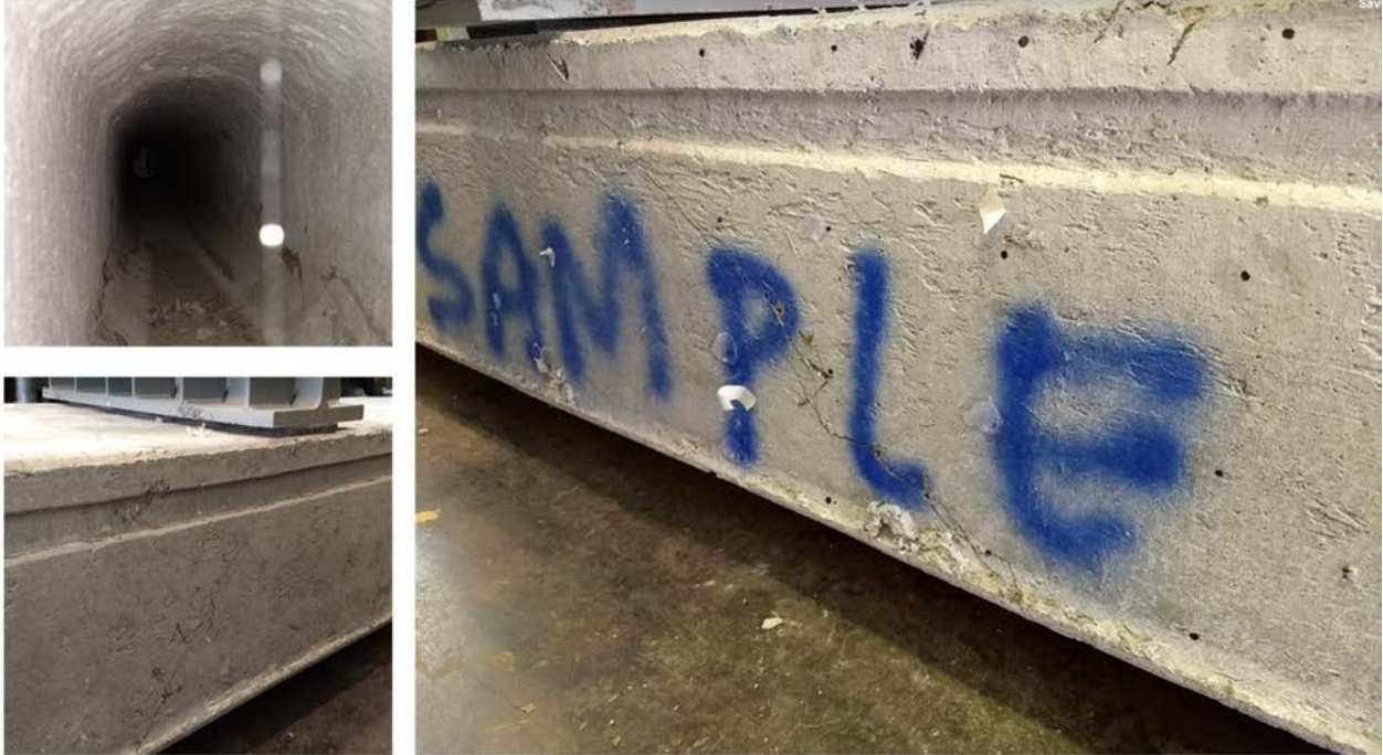
Figure B14 - Test span S1-F2-62-3.5
