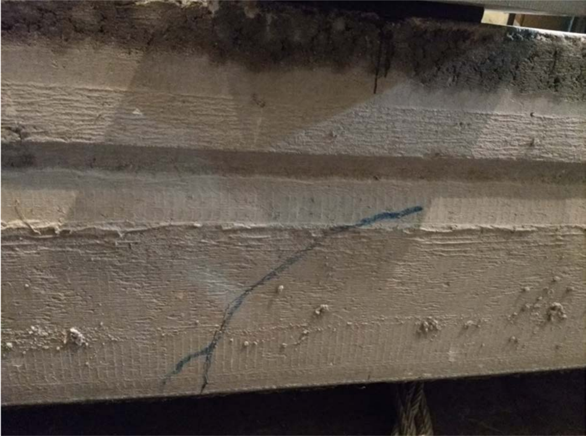
Figure B23 - Test span S2-F1-66-3.0
