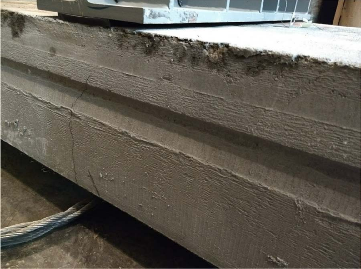
Figure B22 - Test span S2-F1-66-2.8c
