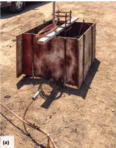
Fig. 7: Embedment of conductors requires close coordination between subtrade contractors: (a) a copper-clad steel ground rod, in the foreground, has been welded to a copper conductor cable that has been pulled through conduit for subsequent encasement in a concrete footing and column (photo courtesy of Mr. Lightning); (b) a copper cable ground loop has been placed in a footing form and routed through a conduit for subsequent connection to a steel column that will serve as a down connector extending to the roof level (photo courtesy of Lightning Protection Systems, Inc. of Tampa); and (c) lighting conductor cables and conduit have been installed along with reinforcing bars, post-tensioning tendons, and electrical conduit in a column joint (photo courtesy of Guardian Lightning Protection)
