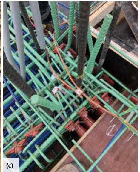
Fig. 7: Embedment of conductors requires close coordination between subtrade contractors: (a) a copper-clad steel ground rod, in the foreground, has been welded to a copper conductor cable that has been pulled through conduit for subsequent encasement in a concrete footing and column (photo courtesy of Mr. Lightning); (b) a copper cable ground loop has been placed in a footing form and routed through a conduit for subsequent connection to a steel column that will serve as a down connector extending to the roof level (photo courtesy of Lightning Protection Systems, Inc. of Tampa); and (c) lighting conductor cables and conduit have been installed along with reinforcing bars, post-tensioning tendons, and electrical conduit in a column joint (photo courtesy of Guardian Lightning Protection)
