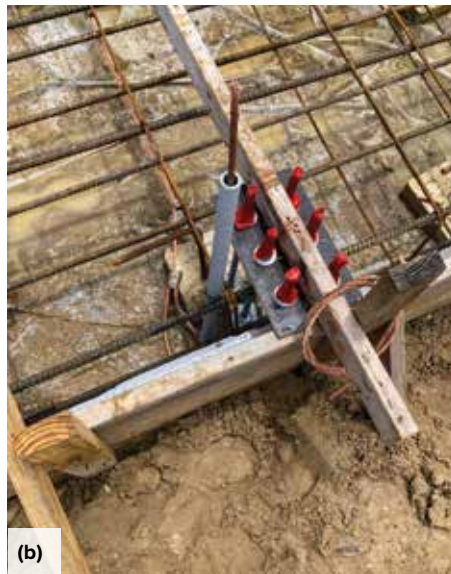
Fig. 7: Embedment of conductors requires close coordination between subtrade contractors: (a) a copper-clad steel ground rod, in the foreground, has been welded to a copper conductor cable that has been pulled through conduit for subsequent encasement in a concrete footing and column (photo courtesy of Mr. Lightning); (b) a copper cable ground loop has been placed in a footing form and routed through a conduit for subsequent connection to a steel column that will serve as a down connector extending to the roof level (photo courtesy of Lightning Protection Systems, Inc. of Tampa); and (c) lighting conductor cables and conduit have been installed along with reinforcing bars, post-tensioning tendons, and electrical conduit in a column joint (photo courtesy of Guardian Lightning Protection)
