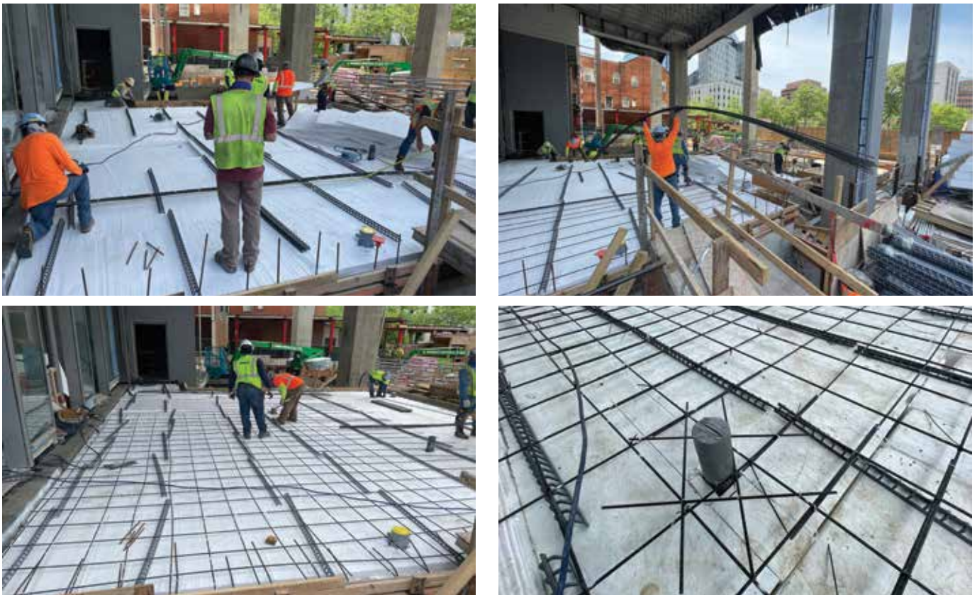
Fig. 4: Installation of No. 3 BFRP reinforcement for one of the topping slabs
