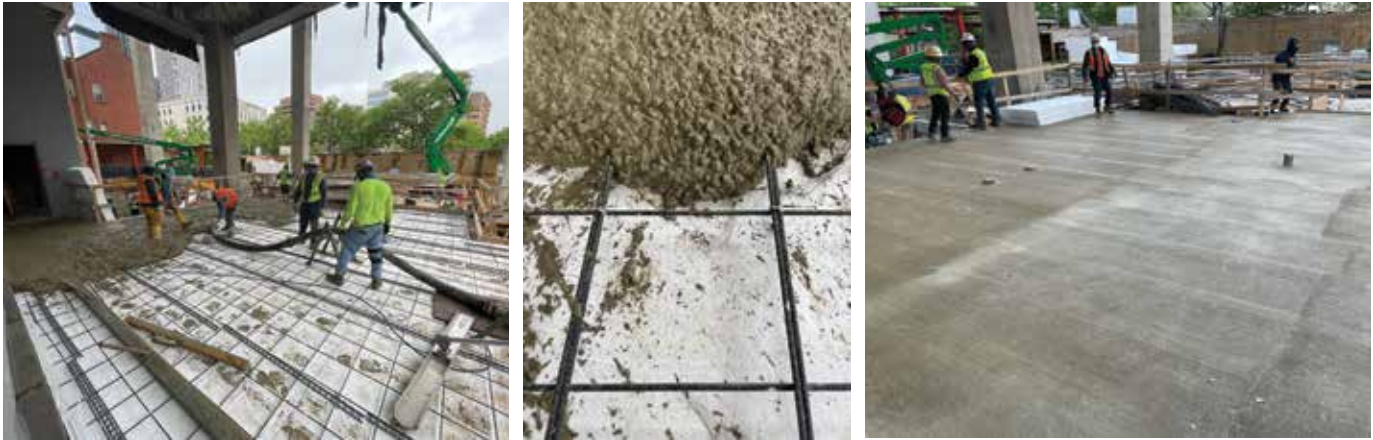
Fig. 5: Concrete placement for one of the topping slabs
