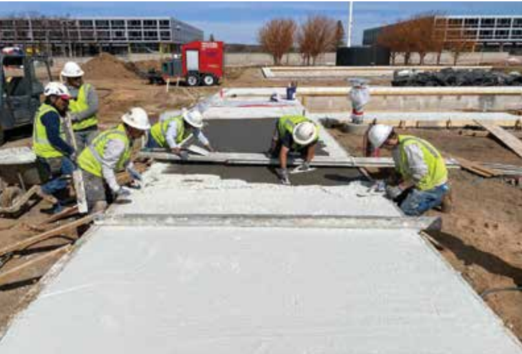
Fig. 3: The careful process of applying white mixture topping to the Air Garden walkways (photo courtesy of Colorado Hardscapes)
