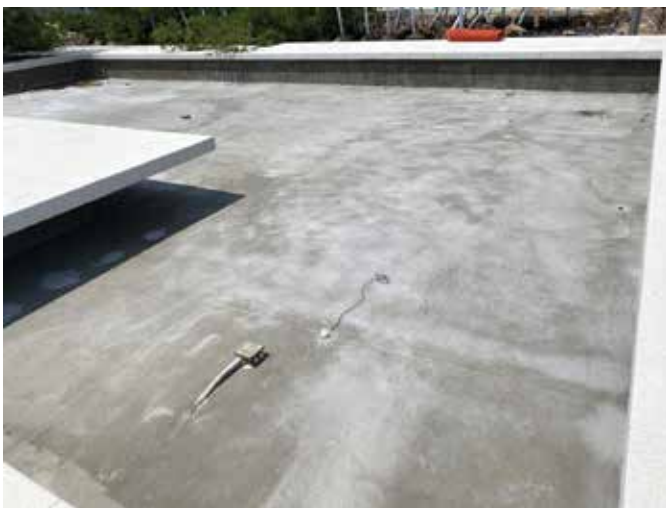
Fig. 2: The mechanical and filtering systems at the bottom of the pool (photo courtesy of Colorado Hardscapes)
