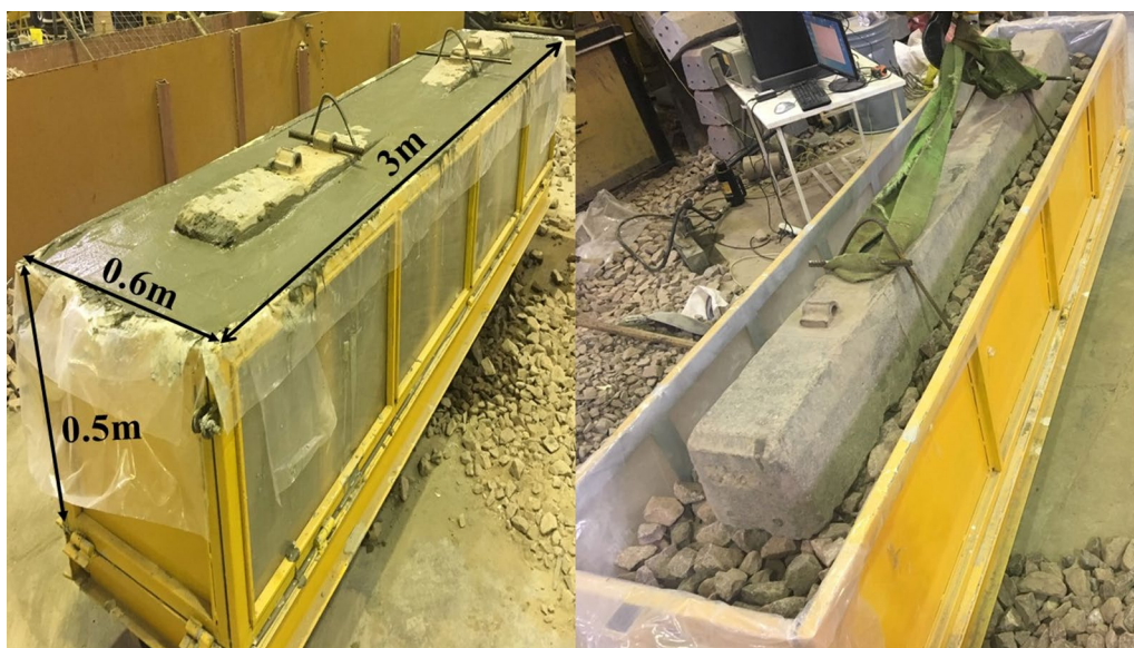
Fig. 5 Casting of PAC beam before and after mortar injection: (Right) before injection, (Left) after injection.
