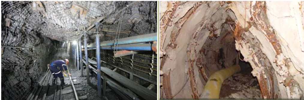
Fig. 1 Rupture-bulking and large deformation of deep surrounding rock.
